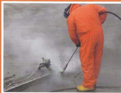
Removing concrete.
