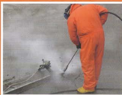
Removing concrete.
