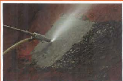
Surface - Sand blasting
