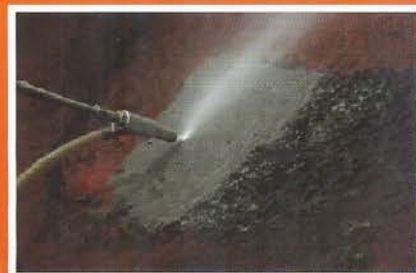
Surface - Sand Blasting
